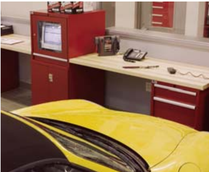
In the service department of Porsche of Nashua, a Lista computer cabinet housing a diagnostic computer teams up with technicians' workstations to make an elegant service bay.
